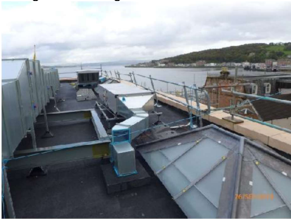
General views: south area looking west.
