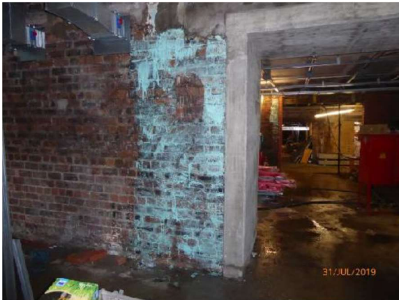
Lower GF Venue: NB: Paint stripper and steam clean in progress to remove the final areas of paint on the Venue brickwork.
