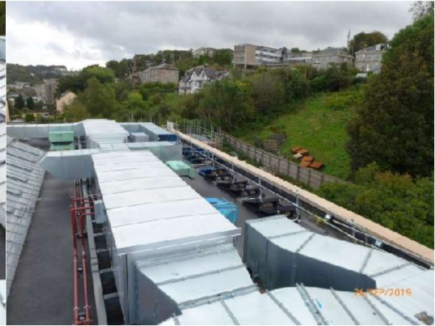
General view: west area looking south.
