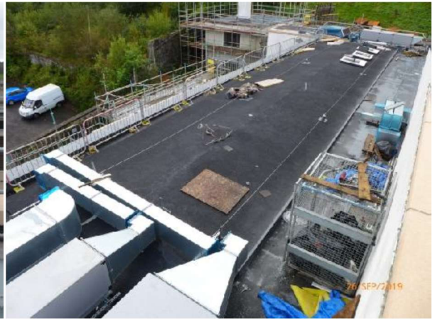
Looking South west: First floor Offices roof– General view.
