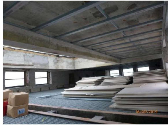
Flytower roof void – floor grillage installation works in progress.
