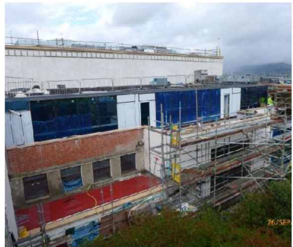
South Elevation – General view.
