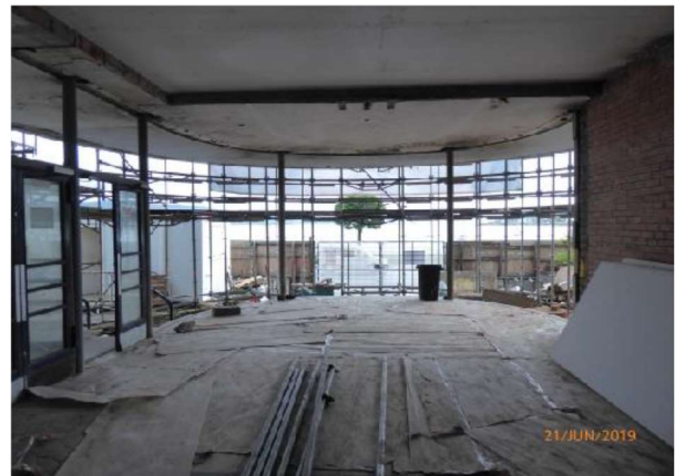
Looking East (Argyle Street): General view of Entrance Lobby.
