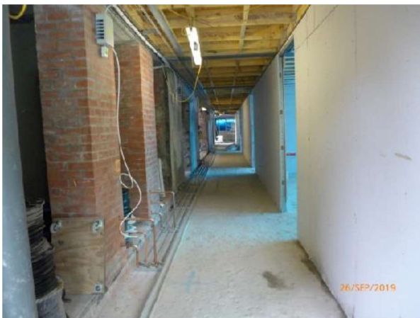
General View of the corridor area behind new offices looking East.
