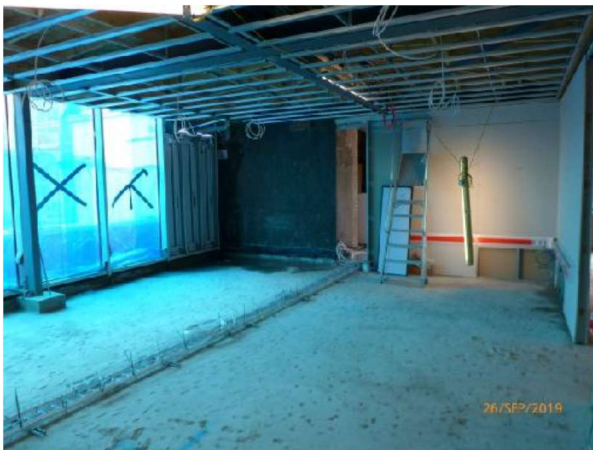
General Views: First Floor: Music Practice Room.
